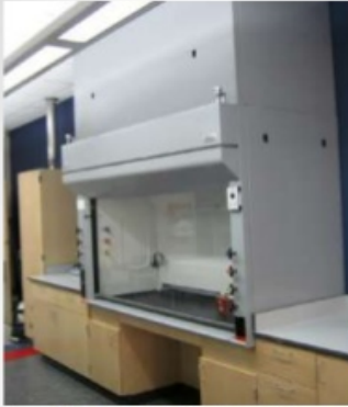
Chemical Fume Hood
