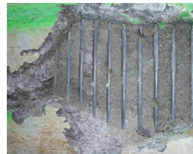
Broken wires – SW Transmission Main
