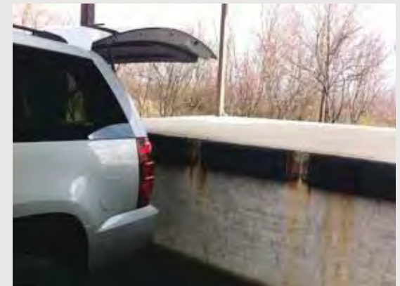
2. The building loading dock was constructed for tractor trailers – not for the types of vehicles used by AL researchers. Vehicle loading and unloading of equipment and gear for field research is difficult due to the configuration of the loading dock and its exposure to the elements.
