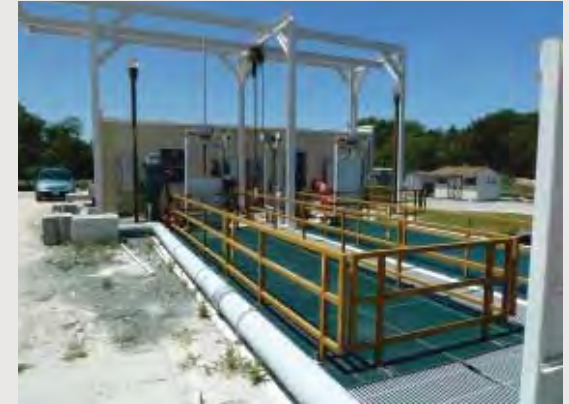
1. Water Pump Station
