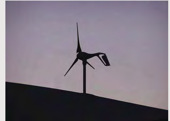
1. Small scale wind turbine
