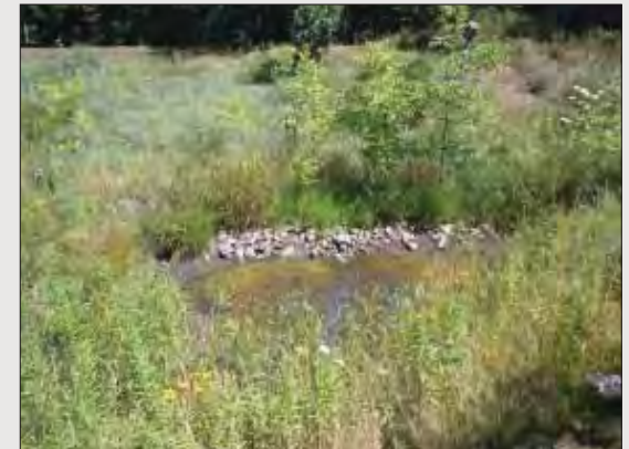
2. Stormwater Collection Pond
