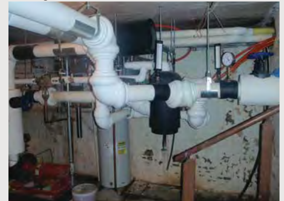
2. Geothermal system at Center Administration
