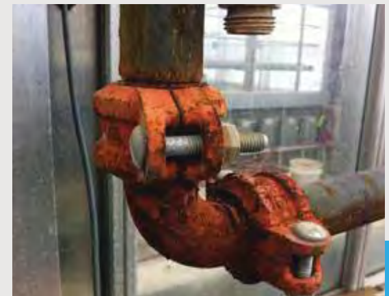
3. AL Greenhouse - Deteriorating plumbing system
