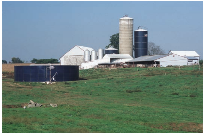
A manure storage tank as part of the conservation plan for a dairy farm in Pennsylvania. During the growing season, stored manure can be applied as fertilizer to soil and used by crops. Photo © Bob Nichols, USDA Natural Resources Conservation Service.
