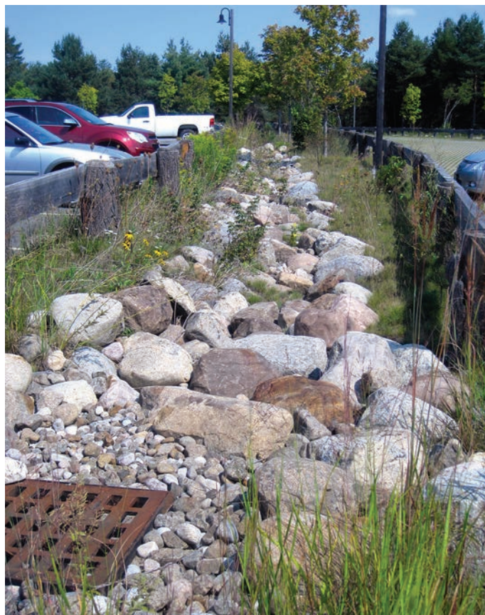
An infiltration trench is a rock-filled trench with no outlet that receives stormwater runoff. Stormwater runoff passes through a combination of pretreatment measures before infiltrating through the soil matrix. Photo © Jane Hawkey, IAN Image Library.
