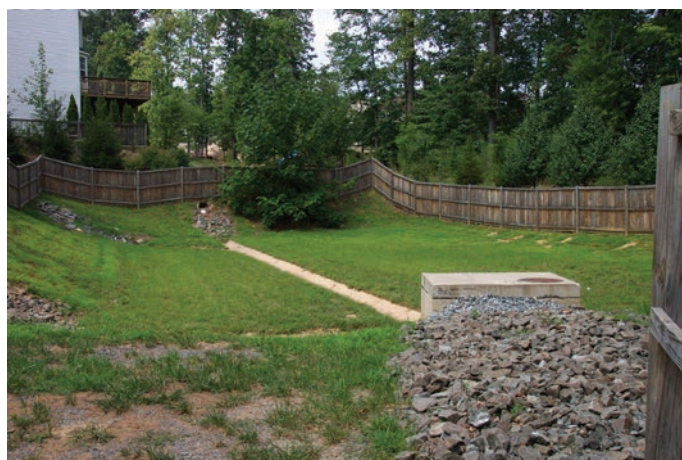
A stormwater drainage basin in a residential backyard directs excess, untreated runoff to the subsurface soil where it can filter naturally through the soil. Photos © Tim Auer, USGS. 68
