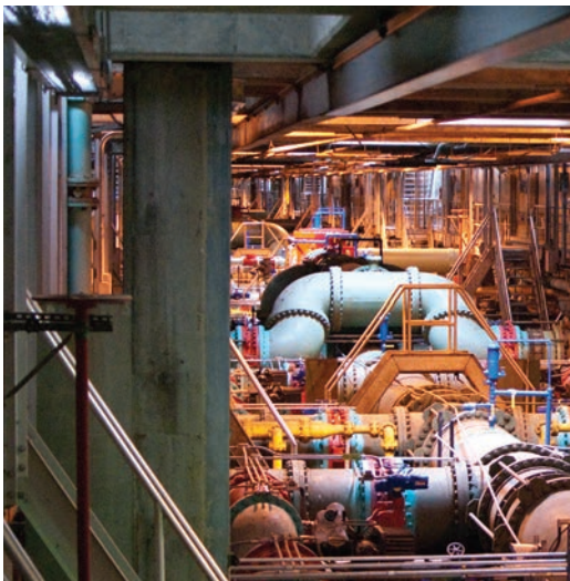
Blue Plains wastewater treatment facility in Washington, D.C. Photo © Chesapeake Bay Program.
