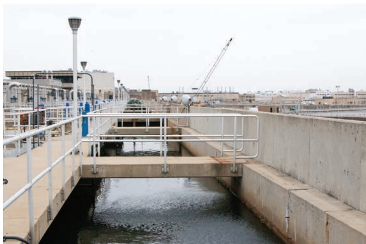
Blue Plains wastewater treatment plant (WWTP) is the largest WWTP servicing the Washington, D.C. metropolitan area. Photo © Chesapeake Bay Program.
