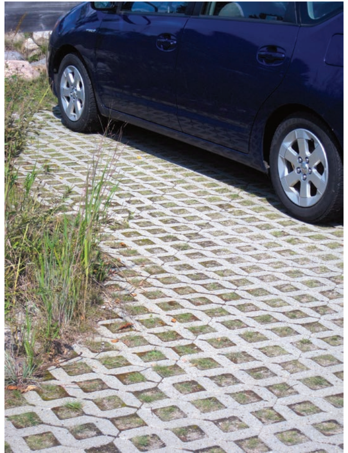
Modular paver blocks serve as a pervious paving system in a parking lot. Pavers fit together like tiles and are set with small gaps between them, creating grooves for water to infiltrate the soil beneath. This practice allows for stormwater to infiltrate into limestone and underlying soils instead of directly into storm sewers. Photo © Jane Hawkey, IAN Image Library.
