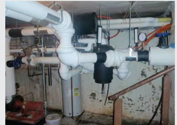
2. Geothermal system at Center Administration
