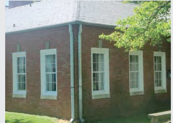
1. New low-E windows were installed in the DuPont building
