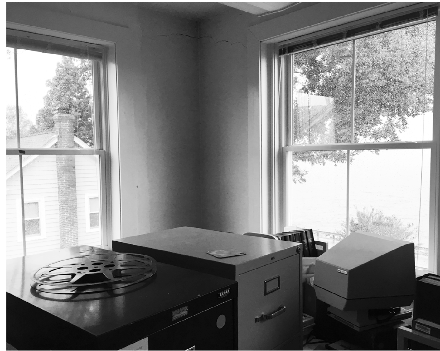
BEAVEN HALL UNDER RENOVATION
