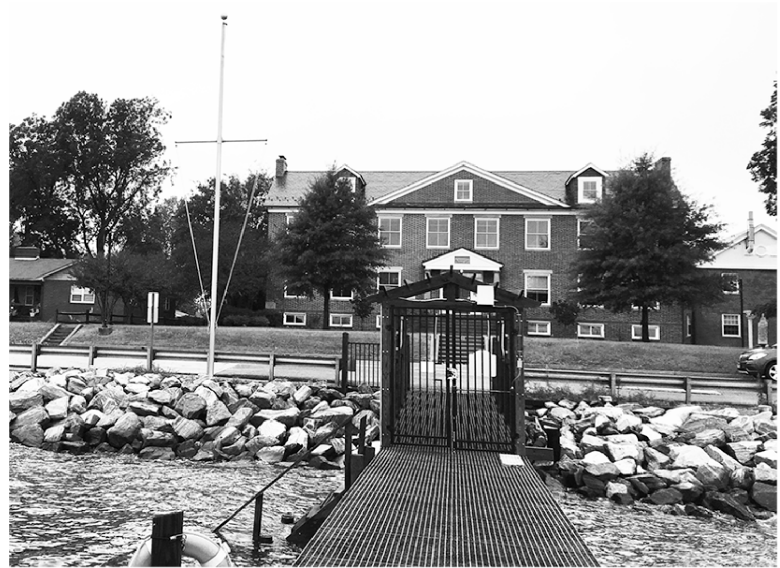
BEAVEN HALL FACADE FROM RESEARCH PIER
