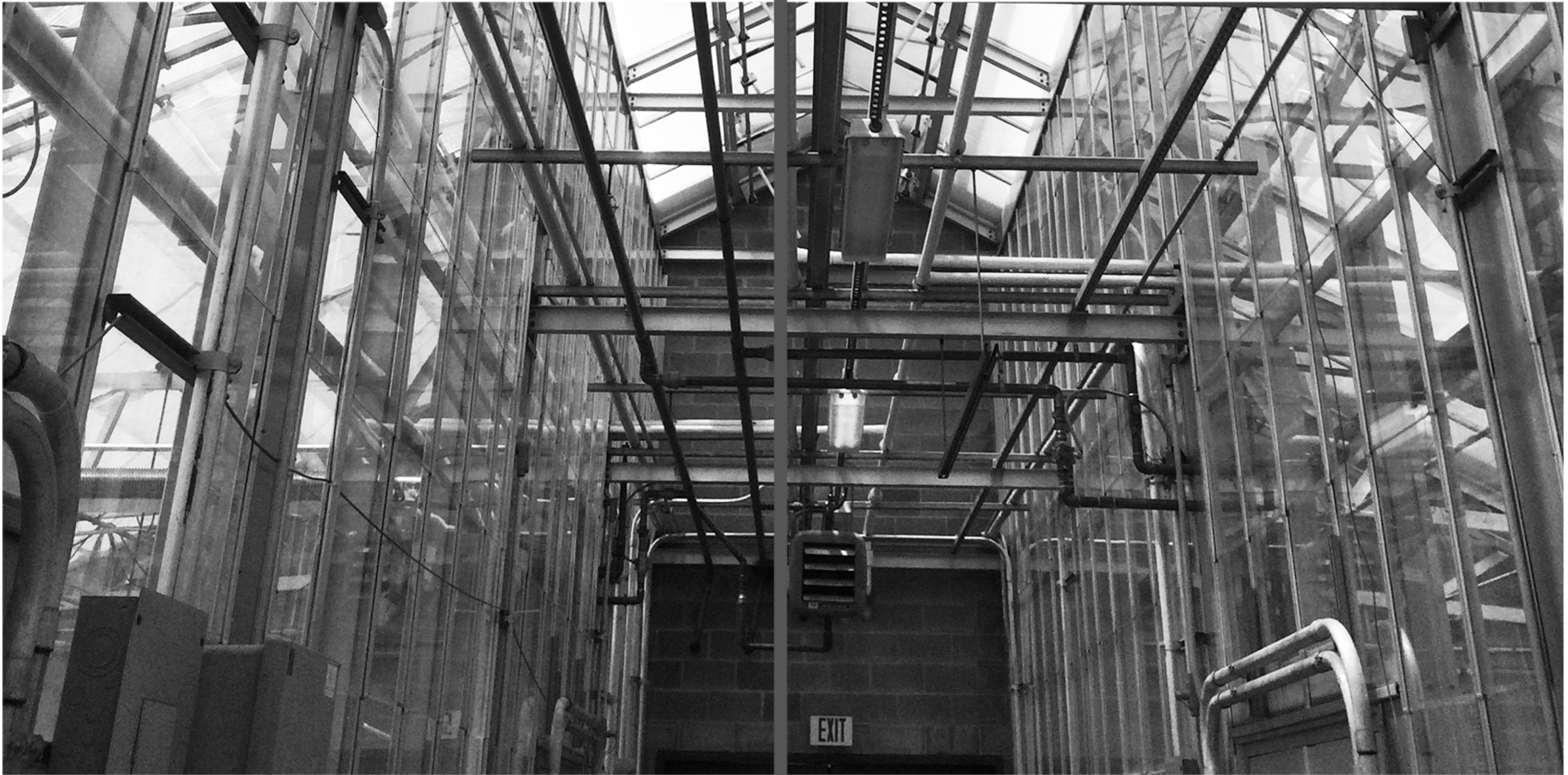
PREREHABILITATION RESEARCH GREEN HOUSE MAIN CORRIDOR
