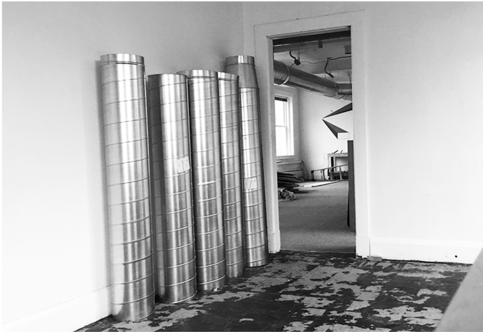
BEAVEN HALL SECOND FLOOR RENOVATION WORK AFTER PARTIAL FLOOR TILE REMEDIATION AND DEMOLITION WORK TO BEGIN
