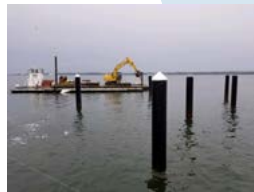
Beginnings of the floating pier repair!
