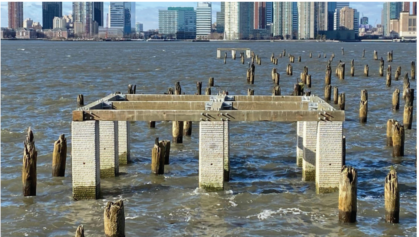
Pier piles retrofitted with textured pile to encourage habitat for oysters in the Hudson River. Photo courtesy of Hudson River Park Trust.
