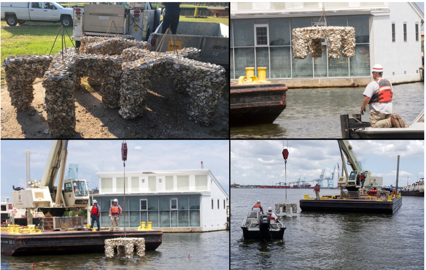
3 ft tall X-Reefs being deployed in Fort Norfolk. Photos courtesy of Russell Burke.
